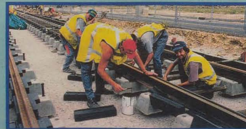
Pose de rails aux Hauts-de-Massane.
